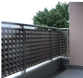
SQB08の施工例の俯瞰
